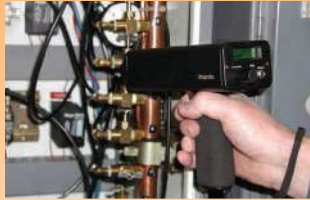
Detect air leaks
