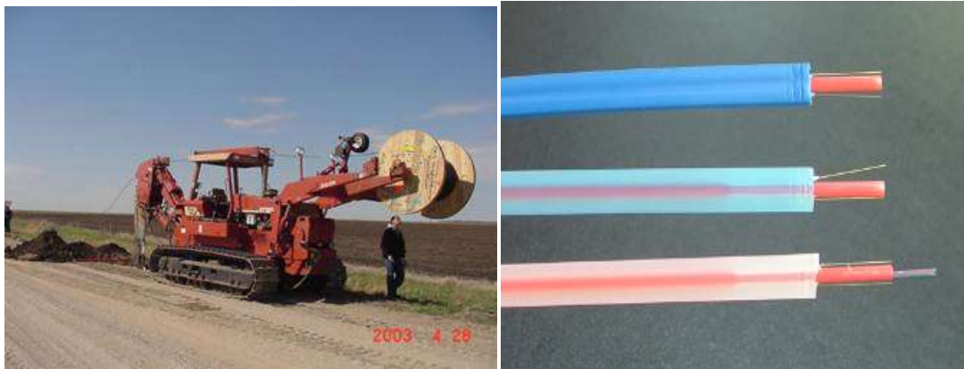
Figure 5: Vibratory plow installation, fiber optic strain and temperature sensing cables.
