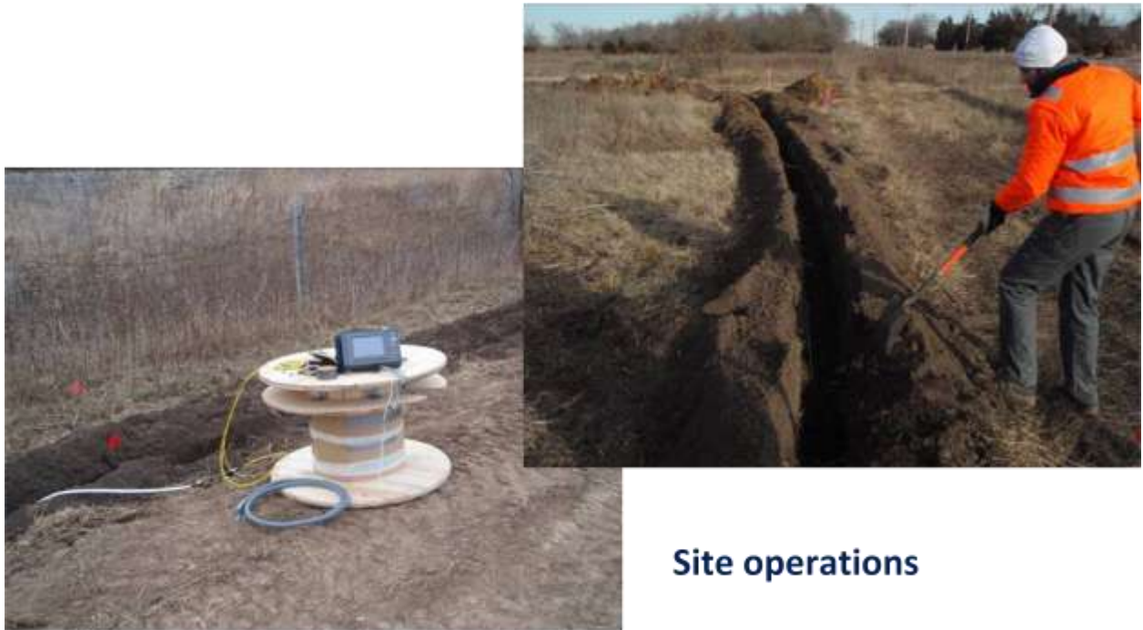
Figure 8 – Onsite sensor verification prior to backfill placement.
